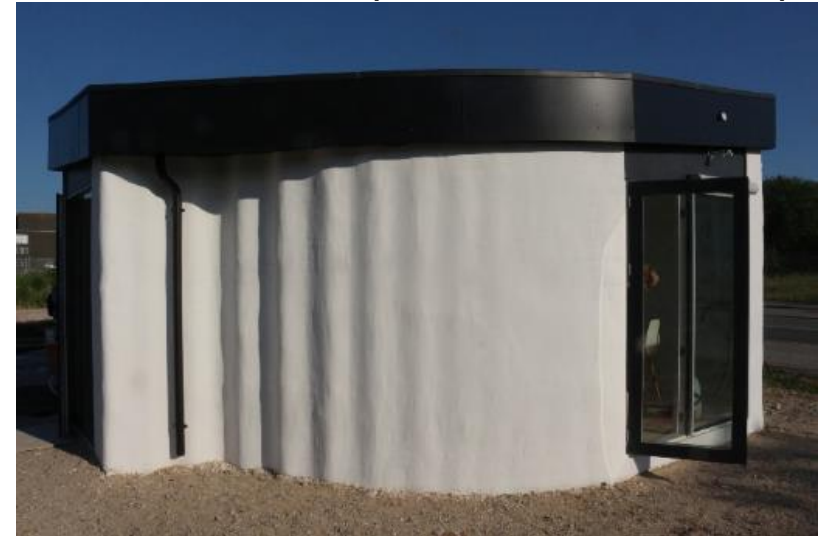
COBOD – first 3D printed house in Europe
